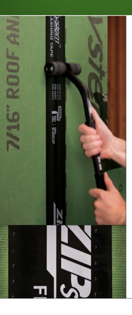
Take the guesswork out of seam sealing with the ZIP System<sup>™</sup> tape roller. Designed to give you a visual indicator where the tape has been rolled, the ZIP System tape roller makes seam sealing simple by leaving a "Z" impression on the tape, for an easy quality control check. Plus, the split-neck roller design allows for easy access in tough-to-reach spots such as inside corners and around windows and doors.
