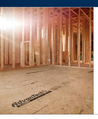
AdvanTech® subflooring is built to a higher standard with published design values above code minimum (PS-2)1 requirements. ESR-1785<sup>2</sup> documents design values for AdvanTech subflooring above commodity-grade panels:
