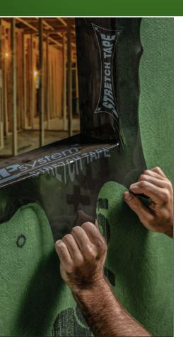
ZIP System<sup>™</sup> stretch tape easily stretches to fit sills, curves and corners with a single piece without having to piece tape segments together. Made of a high-performance composite acrylic, the tape conforms to challenging applications and locks out moisture even over mismatched surfaces.
