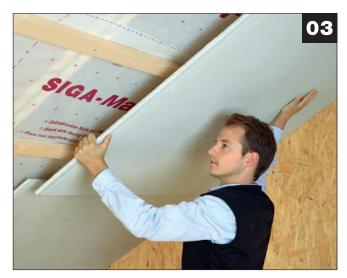
Permanently maintain vapor control layer with mechanical methods, such as battens or interior finish
