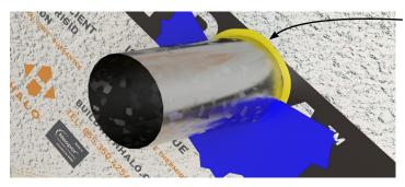
Apply spray foam to fill gaps greater than 1/8" to maintain the continuity of the insulation.
