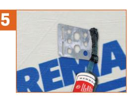
Use SOPRAMASTIC to seal around details, reverse laps and critical areas. For window openings, use a compatible sealant.
