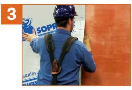
Gradually peel off the remaining silicone release paper, making sure the membrane adheres completely to avoid air pockets and wrinkles.
