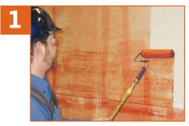
Prime the substrate with SOPRASEAL STICK PRIMER, ELASTOCOL STICK ZERO or ELASTOCOL STICK  $H_2O$ .
