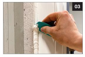
Remove / smooth out excess sealant with caulking tool
