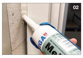
Apply Meltell generously on sealant backer support in window connection joint
