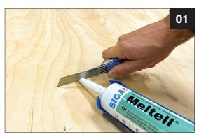
Cut sealant nozzle at a 45 degree angle to approximate joint width
