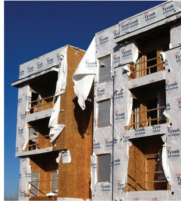
In the event that the housewrap layer is compromised all underlying sheathing could then be exposed to moisture.
