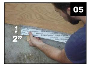
Install Wigluv 100 or wider, minimum 2" onto concrete
