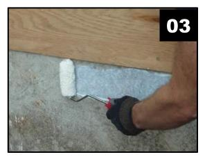
Apply an even coat to masonry using roller or brush
