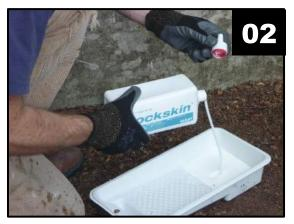
• Shake well and fully unscrew cap to pour Dockskin directly into paint tray
