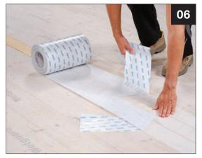
Seal transitions and panel joints on site using Wetguard 200 SA 15" roll or wider All SIGA products are backed by a 10-Year Limited Warranty. Refer to siga.swiss for complete details. We want you to maximize SIGA's performance potential on your project. Contact one of our Application Advisors for support, from architectural detail review to jobsite training for installers.
