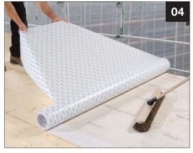
• Gradually remove backing while pressing on using a broom, squeegee, or J-Roller
