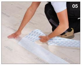
Apply next course with a minimum overlap of 4". Use split backing for easy alignment
