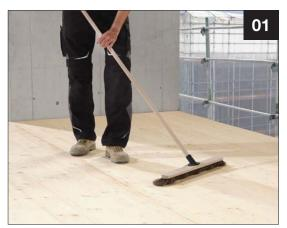
Clean wood surface from dust and loose material
