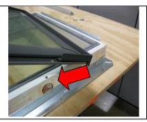
The new pane assembly is ready for replacement and removal of the damaged pane assembly can begin.
