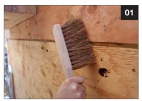
• Clean substrate from dust and excess moisture, make sure nails are driven flush
