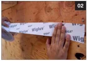
• Apply Wigluv 60 along sheathing joints while ensuring a centered application
