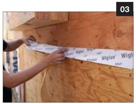
• Ensure at least 1" adhesion on each side of the sheathing. For wider joints and corner details use Wigluv 100.
