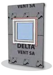
Install DELTA®-MULTI-BAND tape at window edges starting with jamb to ensure proper lapping. Do not tape at window sill to allow for drainage.
